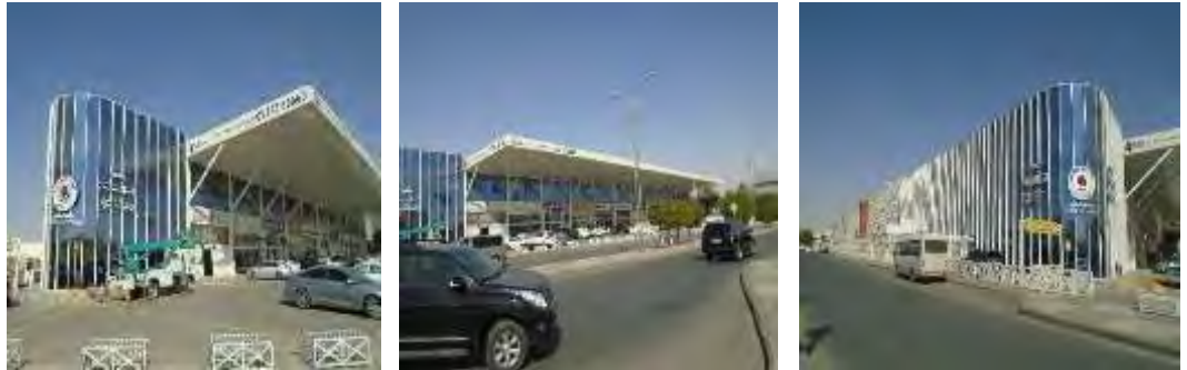
Property No. 1 - Residential / Commercial / Offices, Al Ma'ather, Riyadh
